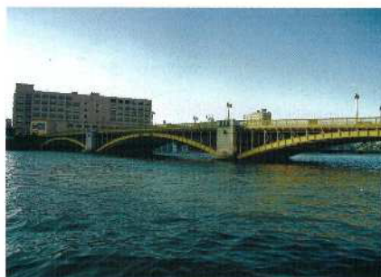
23 蔵前橋 Kuramae Bridge
