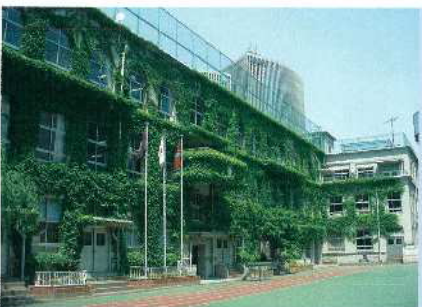
20 中央区立泰明小学校 Taimei Elementary School
